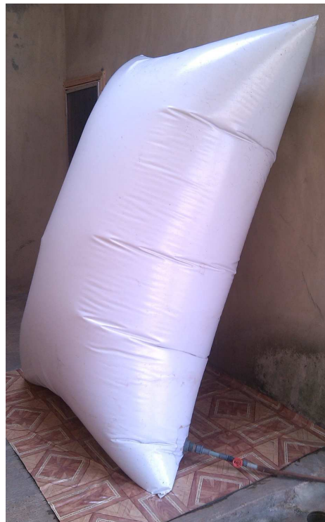
Fig. 1.4: Pillow-shaped airbag for storing the biogas produced.
